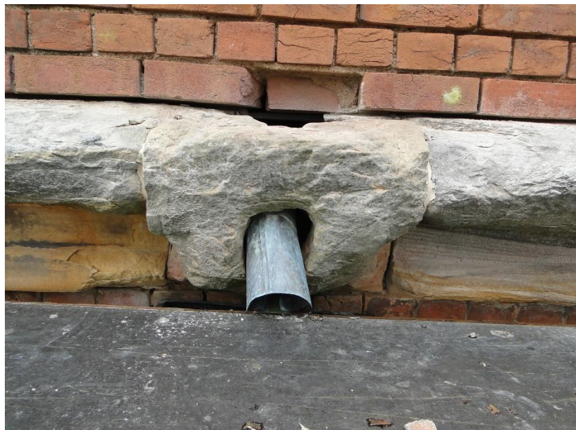
The gargoyle prior to restoration
