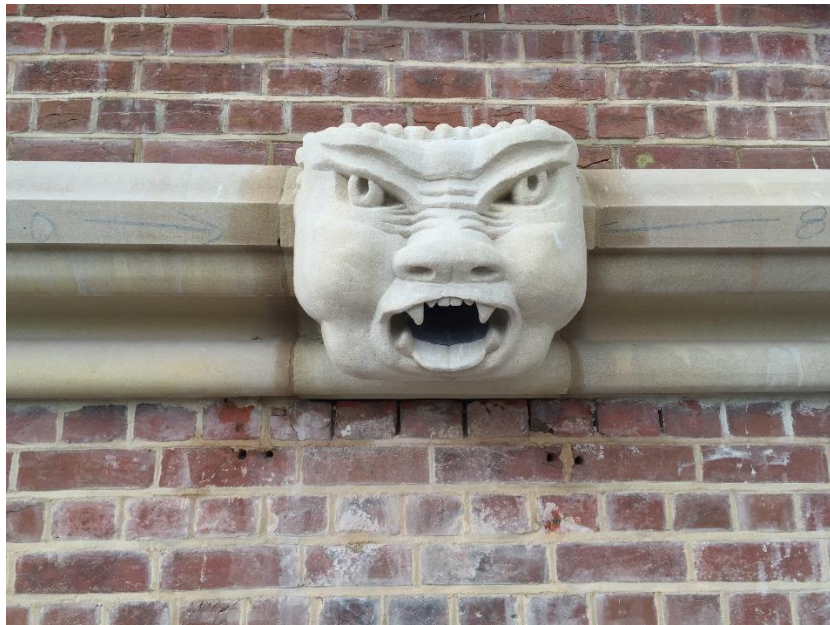
The newly restored gargoyle
